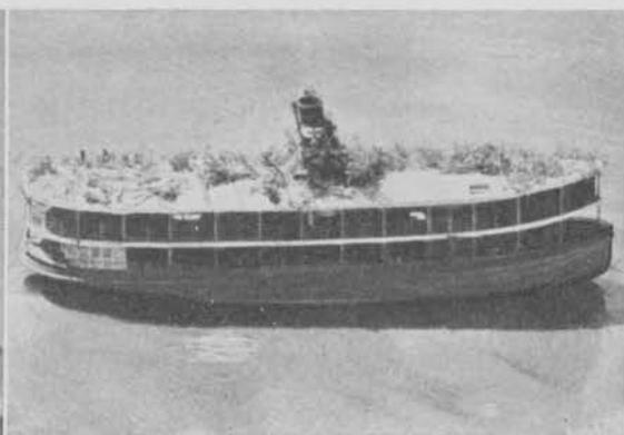
These vessels are small river steamers ranging upwards from 100' over all, with two or more passenger decks. The above photographs show typical creek steamers found in the Burma area.
