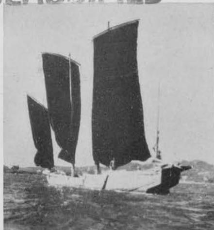
These PECHILI types represent the larger seagoing trading junks; range from 140' to 180' over all, 20' to 30' in beam, and up to 400 gross tons. Normal crews consist of 20 to 30 men. These junks have been extensively used for military transport all along the China Coast.
