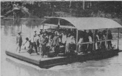
*Right*—Typical native-built car ferry with a capacity of six automobiles unloaded over one of four ramps. The ferry is pulled across the river by a submarine cable, with a gearing mechanism driven by a small gas engine. It is also connected to an overhead auxiliary cable for emergencies.
