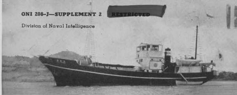
▲ A typical small coastal trawler of 80 to 100 gross tons. Notice that it repeats most of the "large trawler" appearance characteristics.
