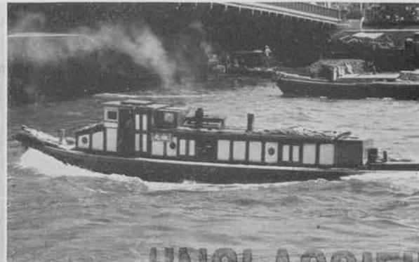
A typical locally built, gas-powered combination house-boat-work launch, used to tow junks, barges, etc. ▼
