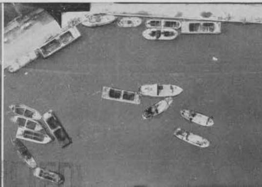
A large 150' x 36' barge used by the Japanese at Wake for banking sludge and coral in connection with a bucket dredge.
