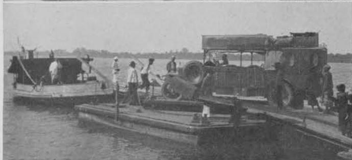
In parts of Indo-China certain "baes" (ferries) are made of specially built shallow barges which are either towed across streams by a cable or poled across. Ramps for landing are bolted in place at the dock.
