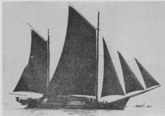
The TONGKANG is a 90' to 100' timber-carrying type with a ketch rig of 3 headsails and loosely footed mainsails.
